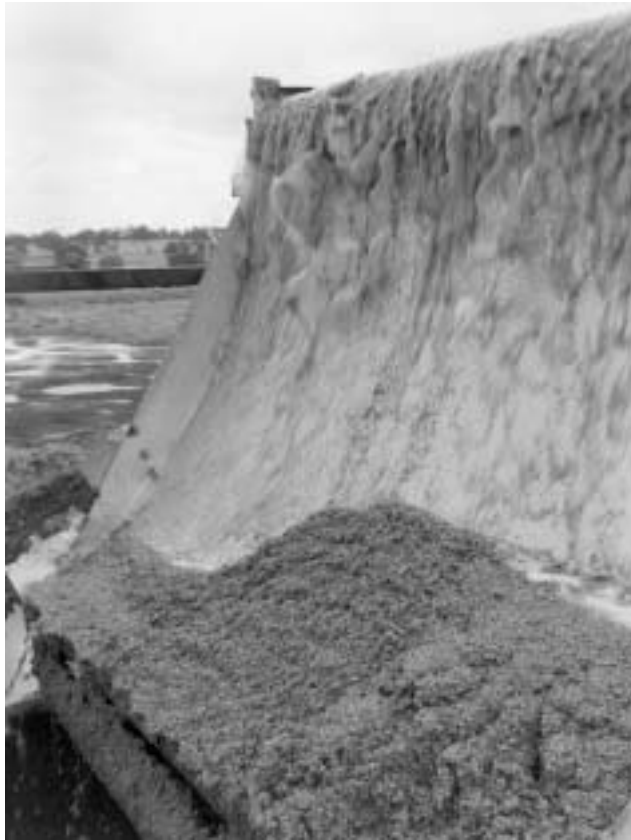
Figure 8. Where screening of solids is employed at piggeries, licence conditions may require collection of screenings samples.
