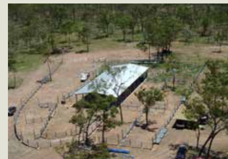
Tank yards under construction, February 2015.
