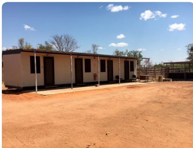
The new office building at the Kununurra quarantine yards
