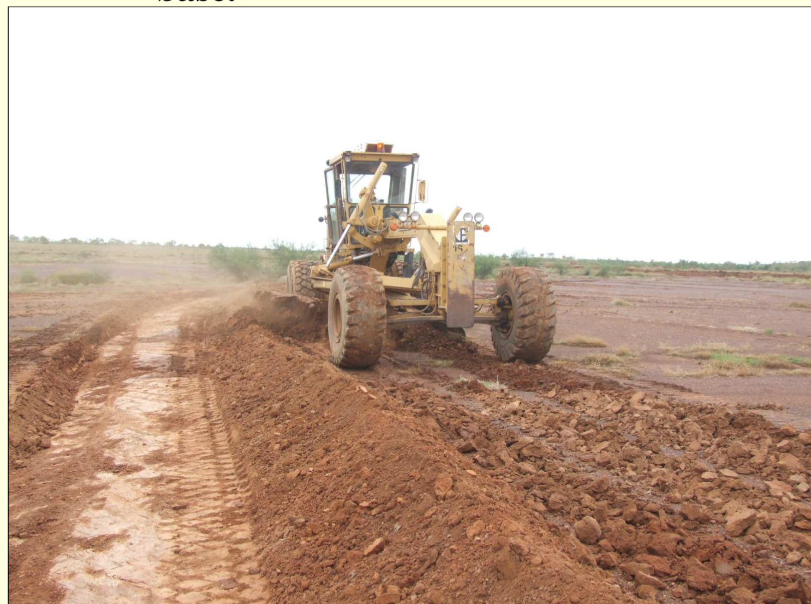
Photo 6. Taking second blade of soil (rolling onto existing bank) on inside of pond.
