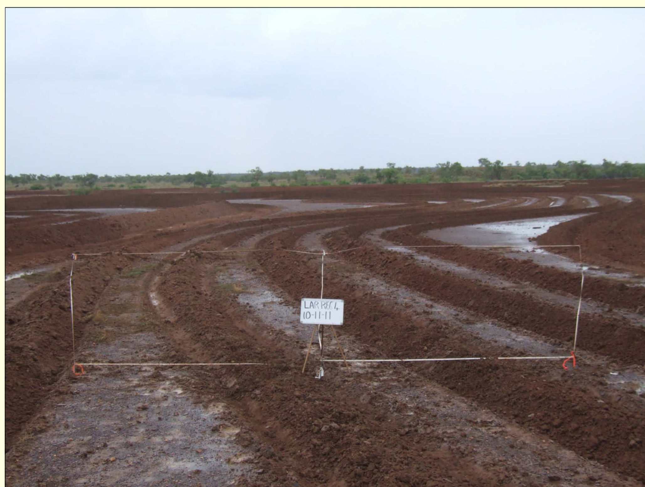
Photo 9. Larrawa station regeneration monitoring site no.4 (post works).
