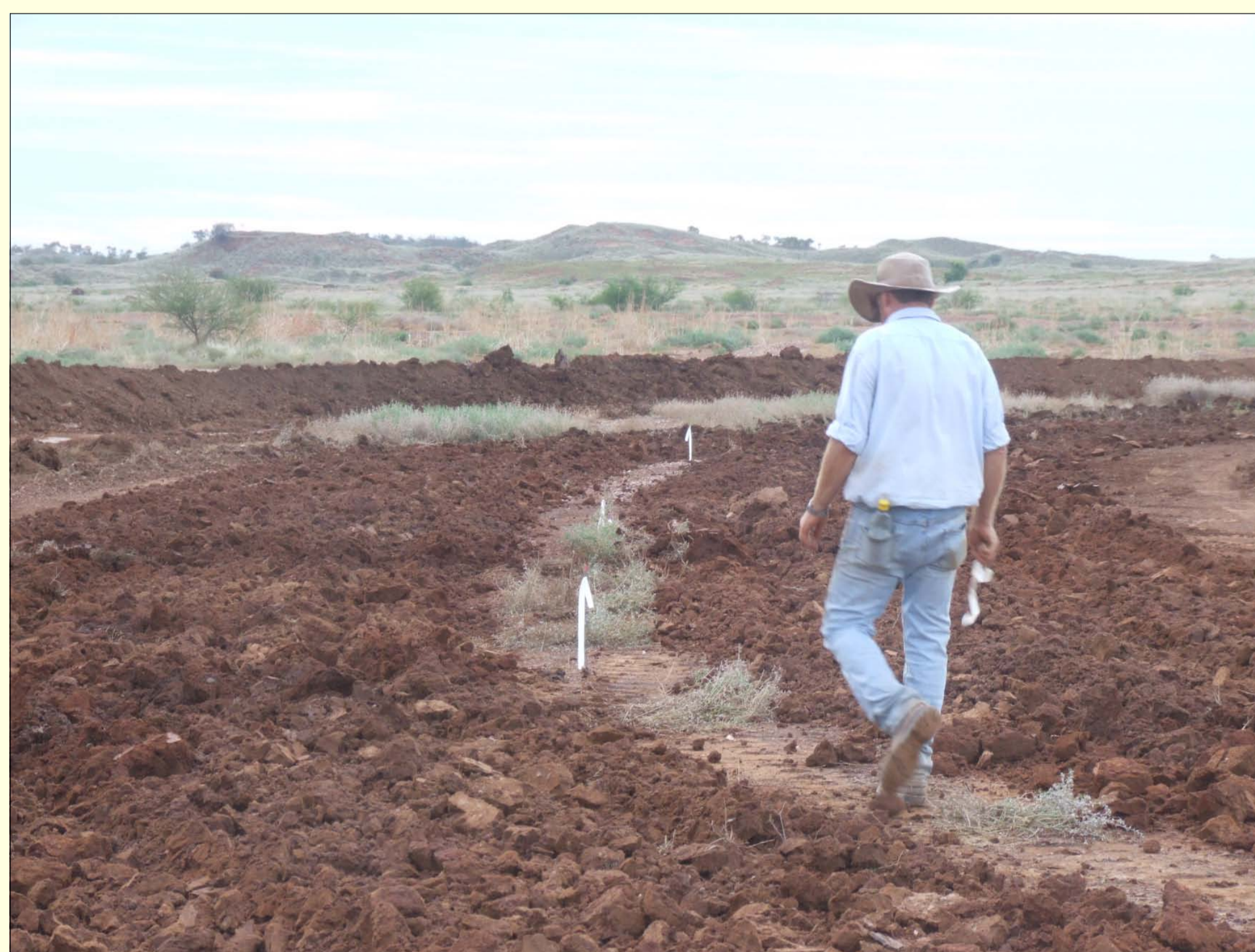
Photo 4. Collecting markers between rip lines before building bank. The non-ripped area between rip lines will form the bank base.
