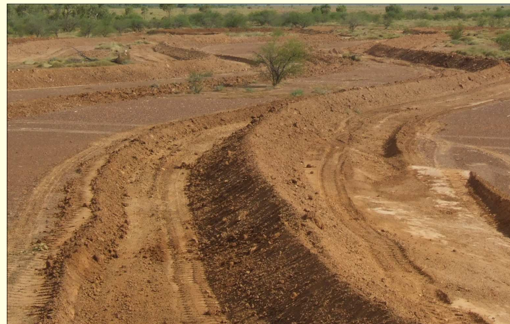
Photo 7. Completed bank. The domed top will allow rainfall to flow away, minimising pooling on bank top.
