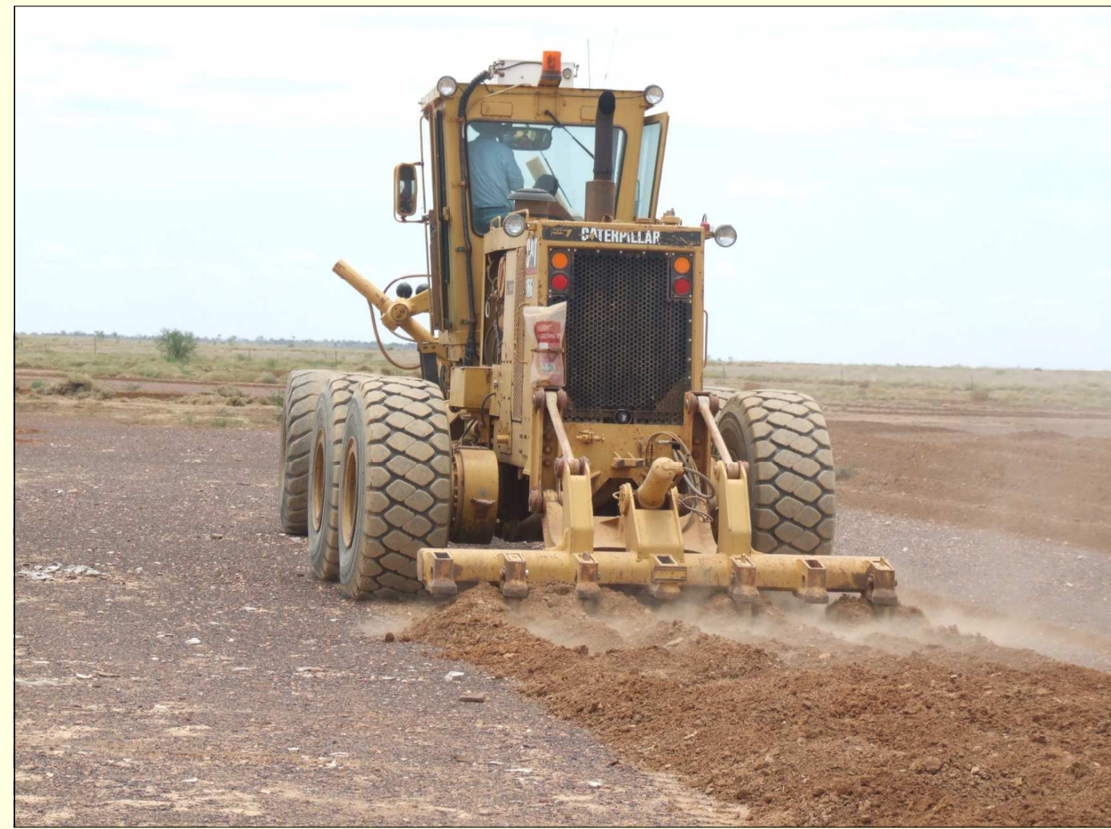
Photo 2. Ripping before bank construction with 16G grader.
