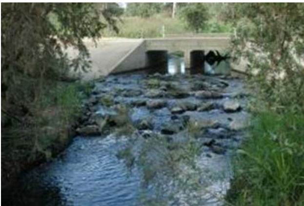
Example of the type of solution to be installed: a rock ramp fishway (Fitzroy Basin Association).
