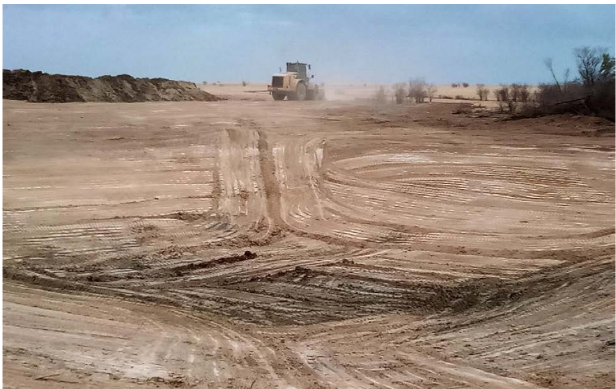
Figure 1. One of Bendemeer's dry dams being cleaned in April 2020.
