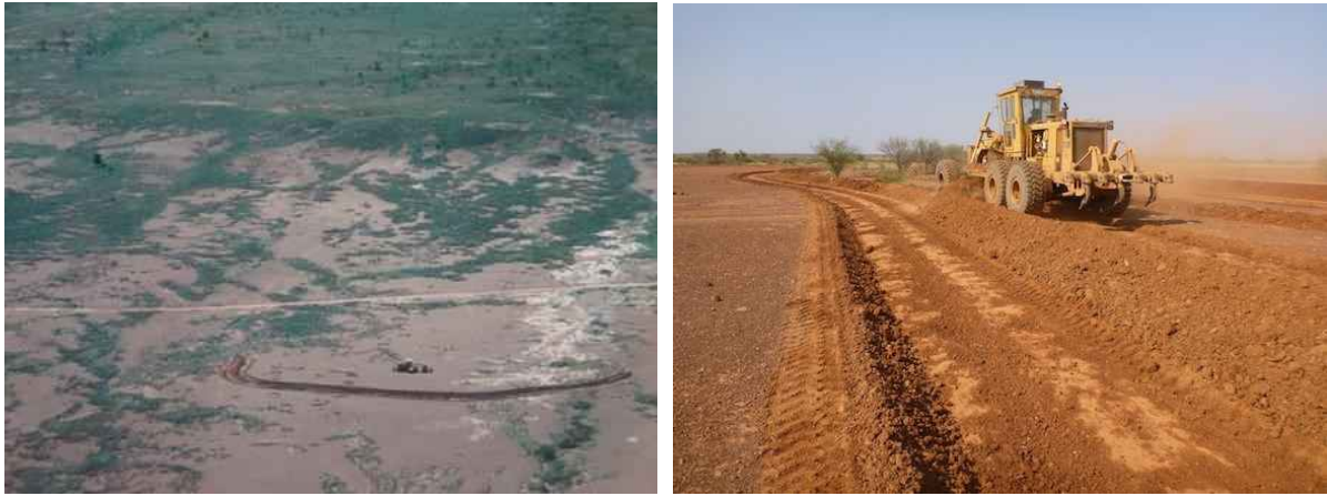
Figure 23. Bank design and construction by professional survey staff and a large grader (Cat G16) is recommended (Photos: Larrawa and Ray Thompson).
