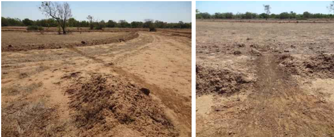
Figure 25. Wallabies are damaging pond banks near the Fitzroy River: L. Wallaby pads over banks across ponds; and R. Degradation of a pond bank ('Go Go' Station) in Sept. 2014.
