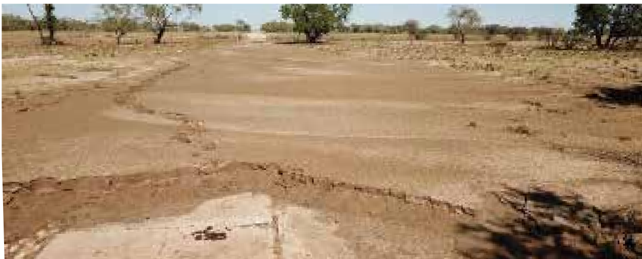
Figure 1: Sediment across the road after the 2019 Monsoonal event
