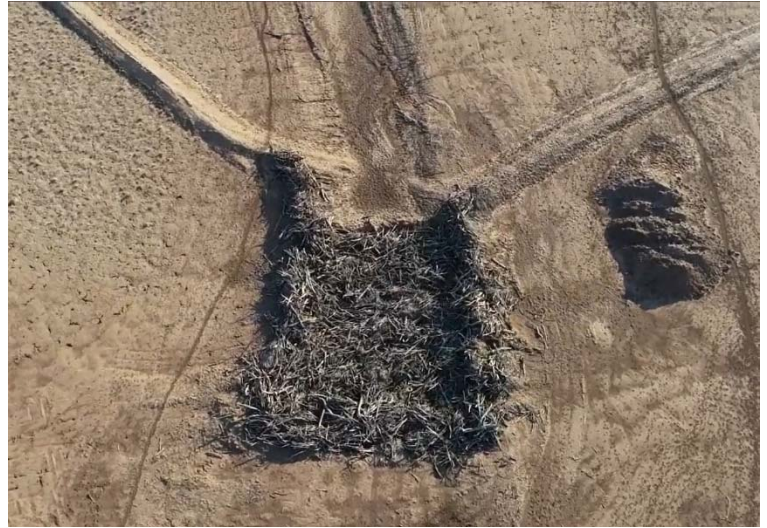
October 2020 – Another leaky barrier further upstream
