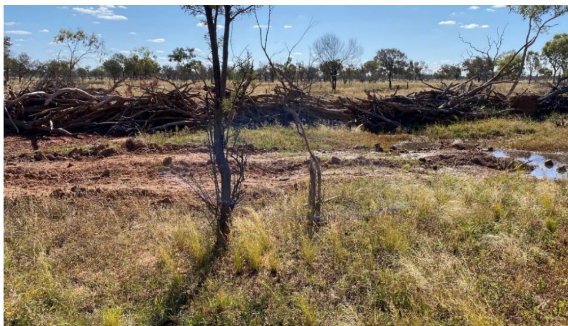
Figure 2: Timber weirs slowing the overland flow, 23/11/2020
