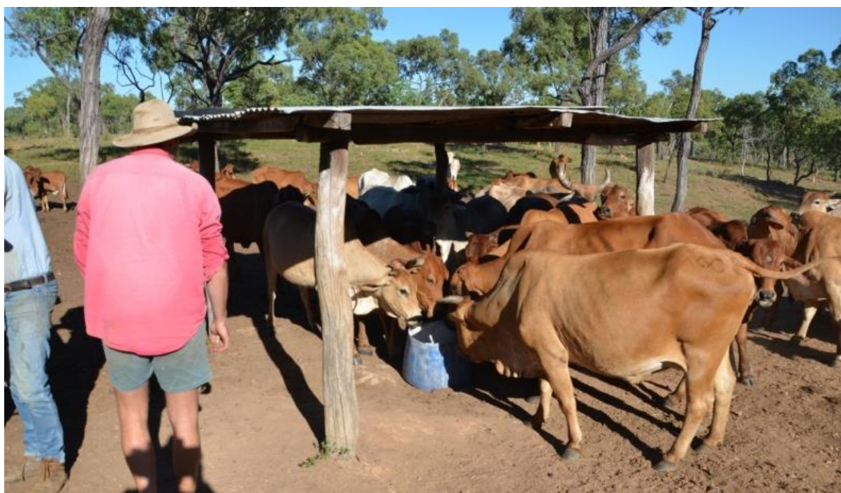
Image 13. Ironwood posts and Leichhardt Pine bearers are used for lick sheds on Karma Waters. Each shed costs around $600, including corrugated iron and labour, when 12 sheds are built at one time.
