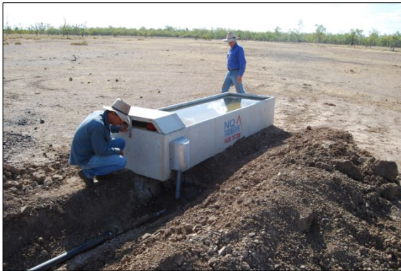
Installing new water infrastructure on Greenhills
