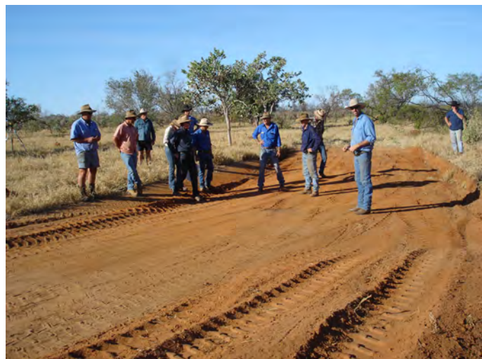
Examining a completed diversion bank at Liveringa station.
