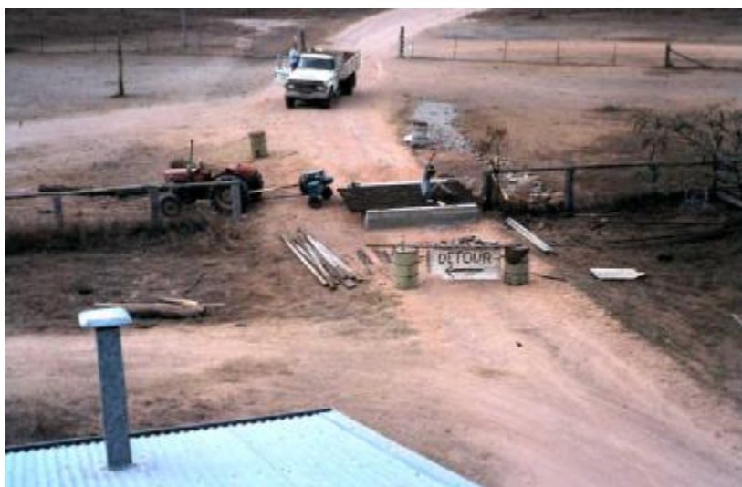
Building a new grid at the main yards, 1976 [Photograph: Mark Savage]
