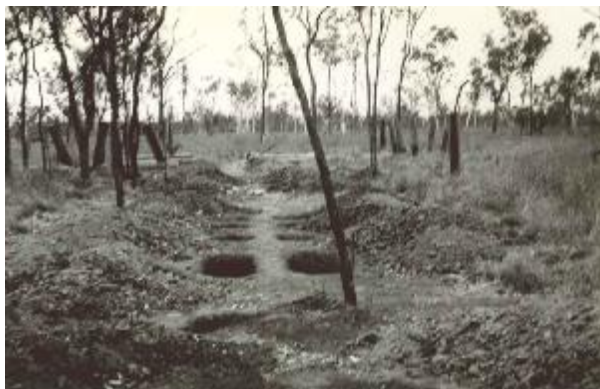
The foundations for the main yards
