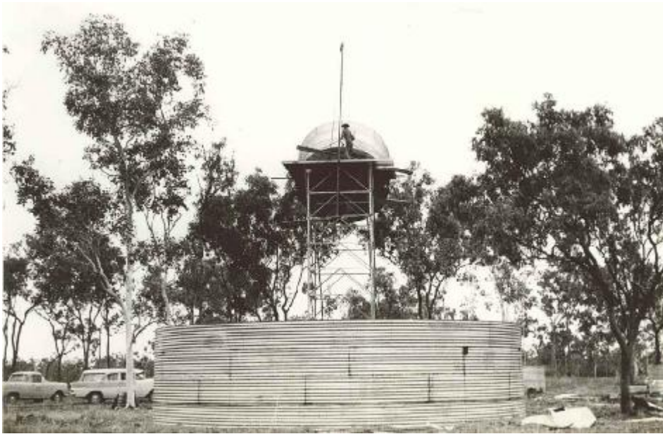
Erecting the high tank at the office circa 1964
