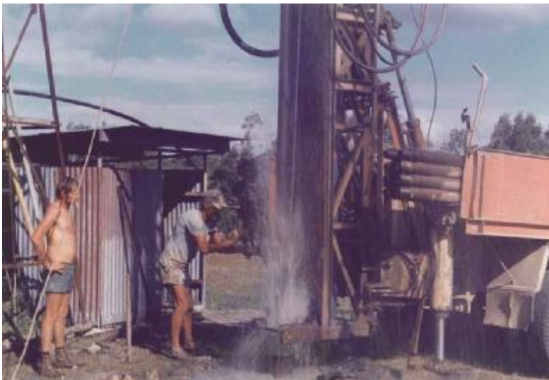
Drilling the new Teddy's Mill bore, May 1988
