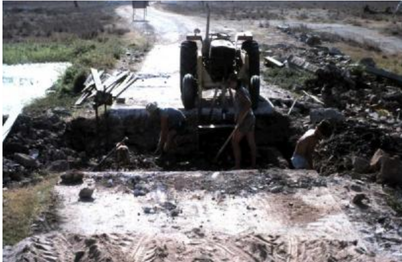
Stan Allan, Peter Dunster and Marcus Platen placing a grid to the lagoon causeway, September 1977 [Photograph: Mark Savage]
