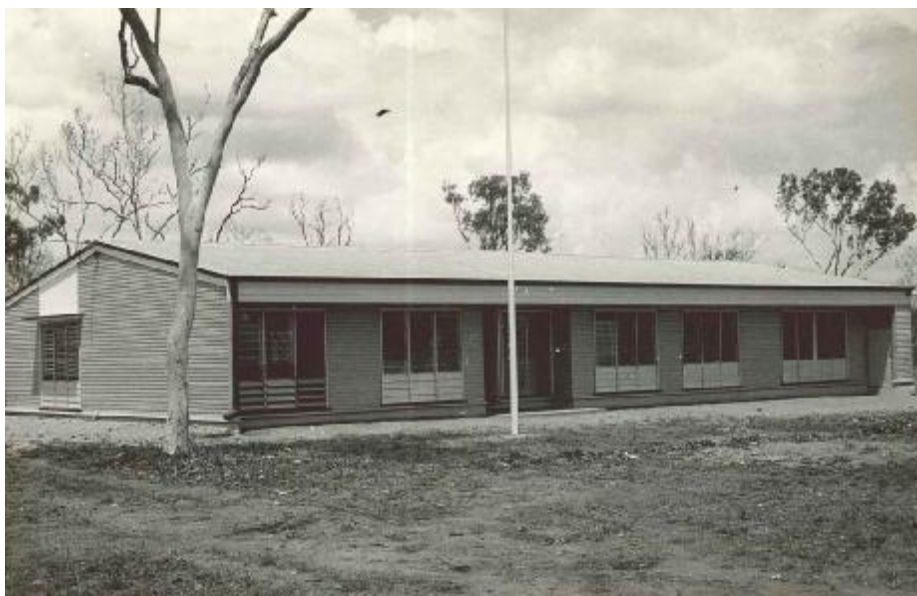
The Swan's Lagoon office on completion, 1965 [Photograph: Rod Strachan]
