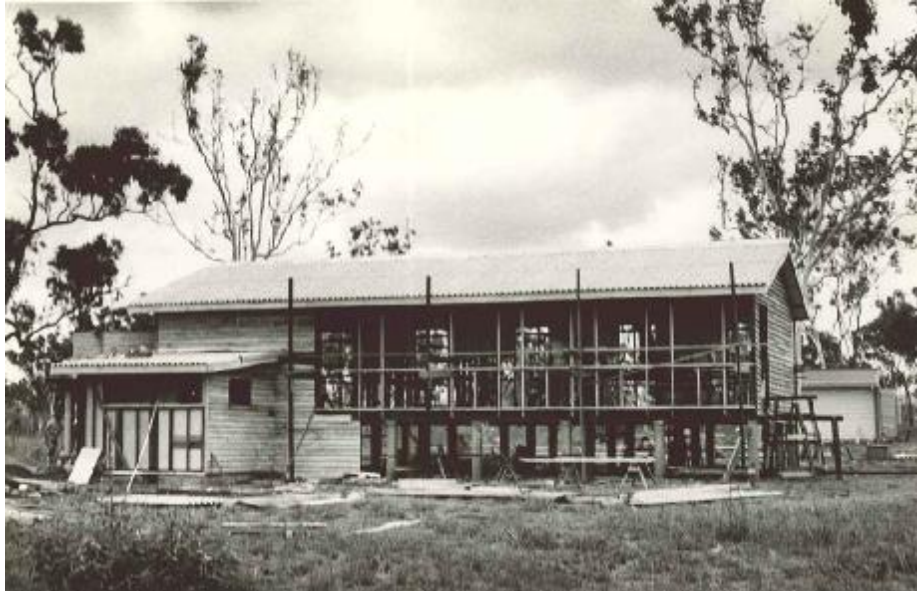
Construction of the first single men's quarters circa 1964 [Photograph: Rod Strachan]
