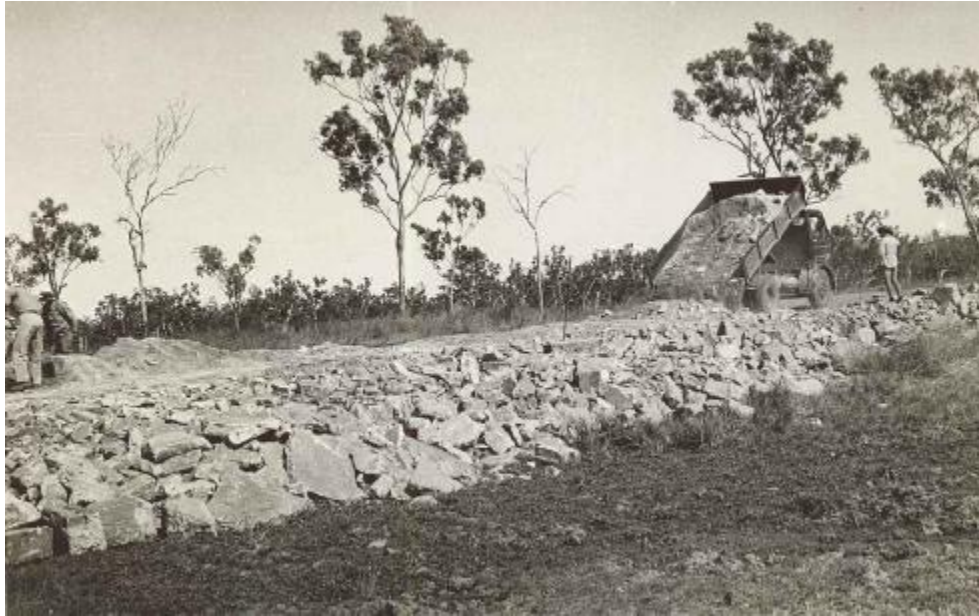
Building the lagoon causeway on the road into Swan's Lagoon circa 1964. The causeway was concreted in 1972.
