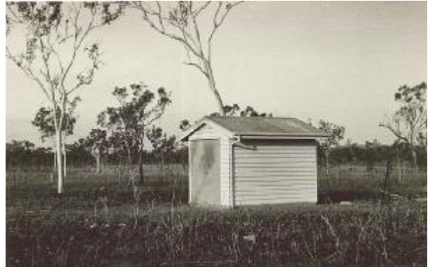
Fuel shed: The first station building erected
