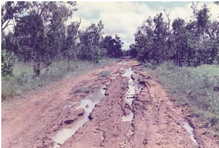
Benjonney road after heavy rain, February 1991 [Photograph: Geoffry Fordyce]
