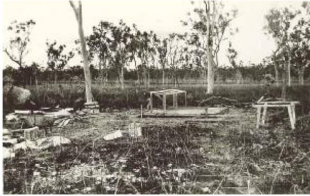
The foundations for the first station building [Photographs: Rod Strachan]
