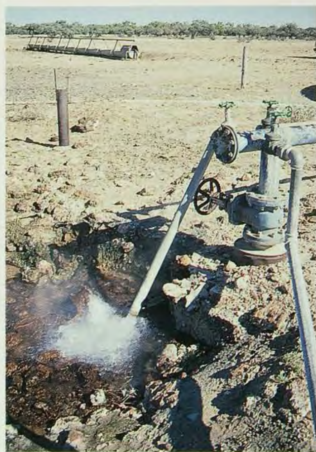
Capped bores conserve water. Piping and troughs allow better distribution of water points.
