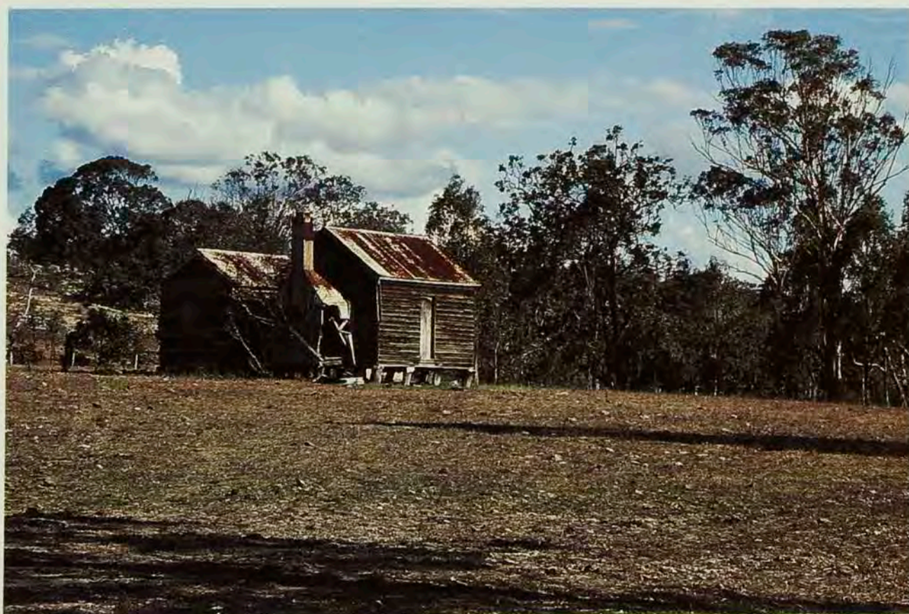
▲ Small property size and high stocking rates can put too much pressure on pasture and occupier!
